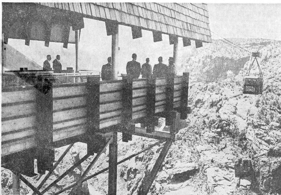
TAKEOFF POINT —Passengers at the tramway loading platform watch the tram, which is painted bright red, approach the north rim of the Royal Gorge. The terminal on the south rim is 119 feet higher than the north rim terminal.
