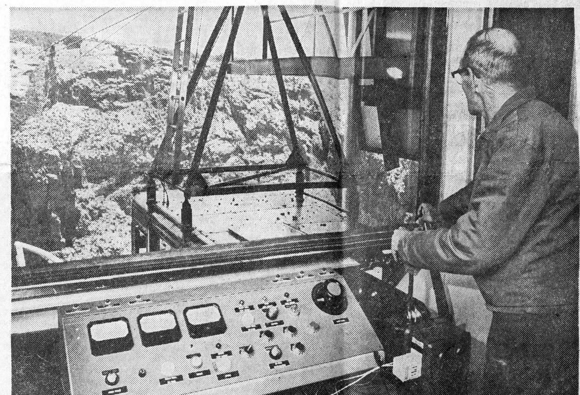
OPERATION CENTER —Ray Matz of Canon City looks out of the control room over the top of the aerial tram, which carries up to 35 persons at a time over the yawning abyss of the Royal Gorge. Matz
